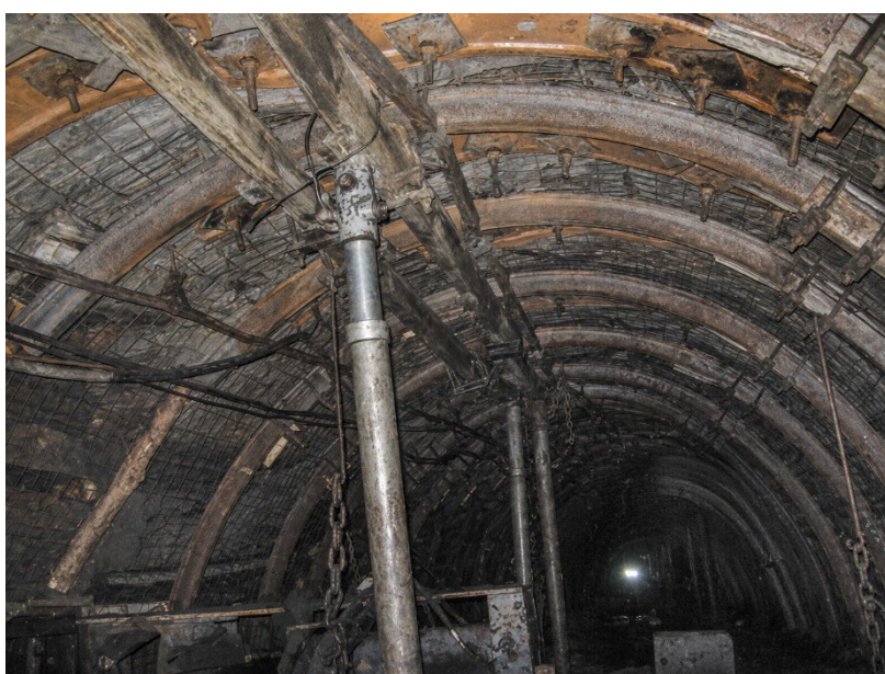
Figure 5. Condition of the 585 collecting roadway at the opening of the first longwall [9]
